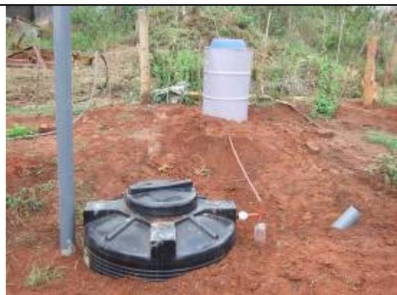
*The 1 m3 biogas system, installed in 2 days. The left feeding pipe still to be shortened, when the concrete at the bottom will have been hardened*
